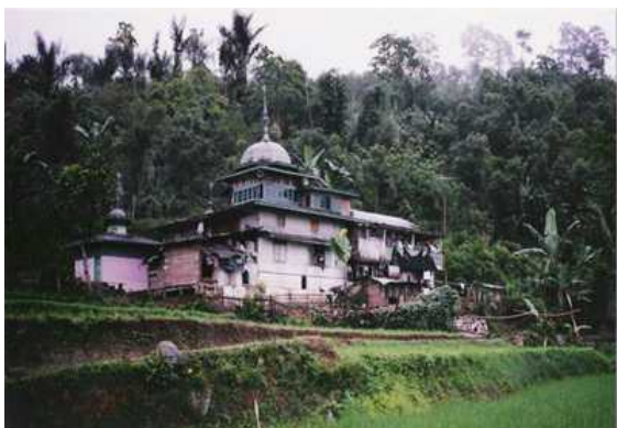
Surau A was built originally in 1918, afterward underwent renovations several times.
